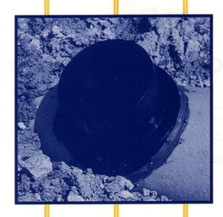
The spigot tap saddle connects the branch branch pipe to the saddle with a flexible coupling. The saddle is bonded to the sewer with epoxy the same as the hub tap saddle.
