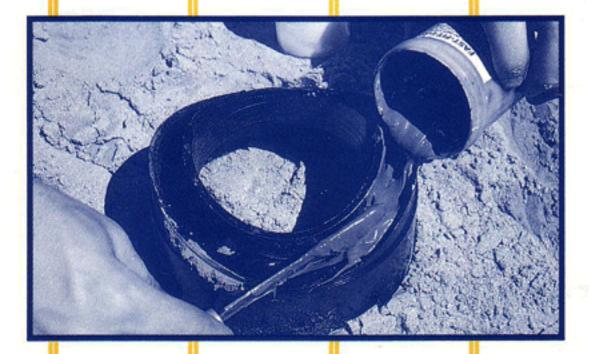
Place mixture evenly into bottom cavity of saddle
