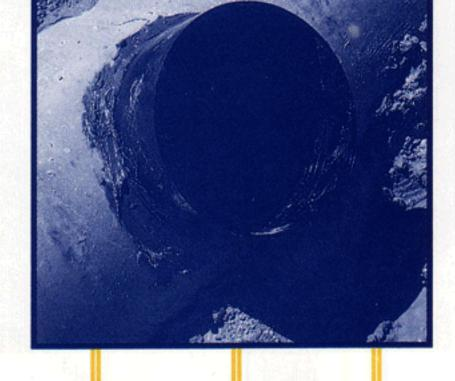
Place hub tap saddle on a clean pipe surface and smooth epoxy around outer edge of saddle. Pipe surface may be wet, but cannot be submerged or have water flowing across joint area.
