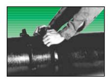
2. Insert the pipe into the socket and press the gasket firmly and evenly into the gasket recess. Keep the joint straight during assembly.
