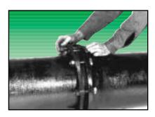
Push the gland toward the socket and center it around the pipe with the gland tip against the gasket. Insert bolts and hand-tighten the nuts. Make deflection after joint assembly but before tightening the bolts.
